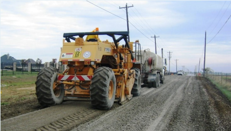
PROJECT PROGRESS IS HERE IN BRENTWOOD PARK
